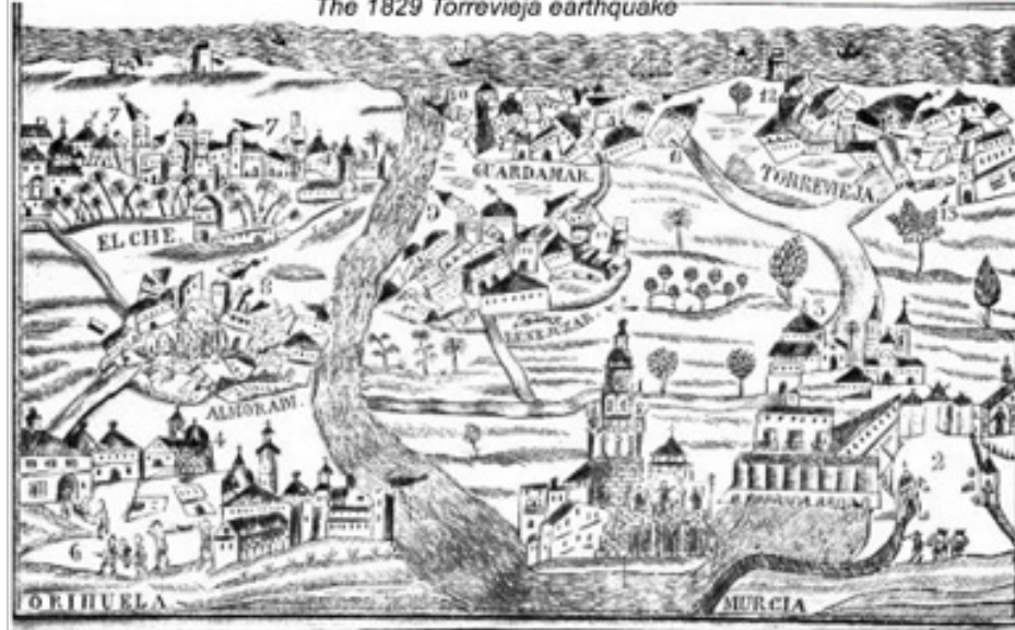
The 1829 Torrevieja earthquake
